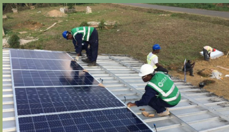
In 2017 CEA designed, procured, and installed a 2.6 kW PV system for an off-grid medical center in Southern Cameroon.
